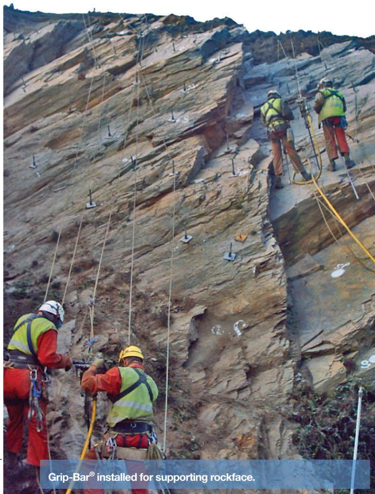
Grip-Bar® installed for supporting rockface.
